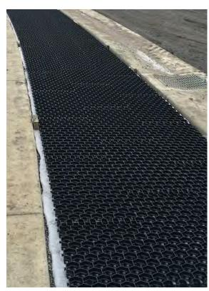
Step 2. If the base is a reactive soil or sand, lay a geofabric over the leveled base before installing an aggregate drainable road base. Lightly compact the site to ensure a level installation of GEOHEX™
